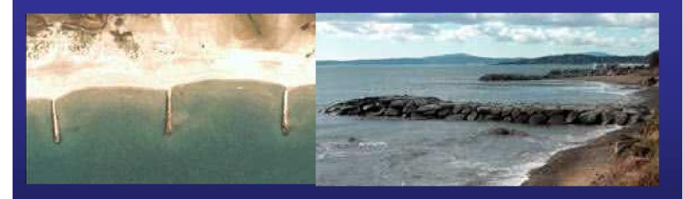
Structured pile of rocks designed to protect the shore against erosion (axis generally perpendicular to the coast).
