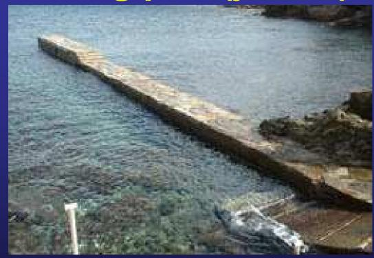
Solid structure with vertical sides (in contrast to rock dump groins) for boats to draw alongside.
